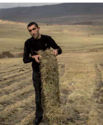
Hand cut grass sods will line the roof borders. Copyright: Tim Flynn Architects
